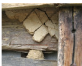
Fmr Castlemaine military quarters_slabs and plaster_Kj_7 Feb 08
