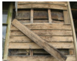
Castlemaine military quarters_slabs under weatherboards_KJ_7 Feb 08
