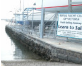
Jacks And McIntosh Boat Repair Facilities Williamstown Aug 2003
