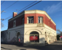
68-70 Armadale Street, Armadale
