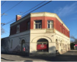
68-70 Armadale Street, Armadale
