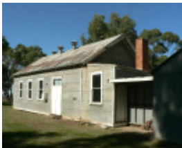
Gringegalgon Soldiers Memorial Hall - viewed from north-west
