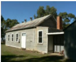
Gringegalgon Soldiers Memorial Hall - viewed from north-west
