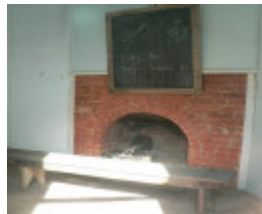
Gringegalgon Soldiers Memorial Hall - rear dressing room
