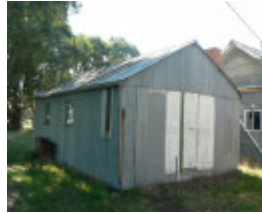
Gringegalgon Soldiers Memorial Hall - supper room/kitchen
