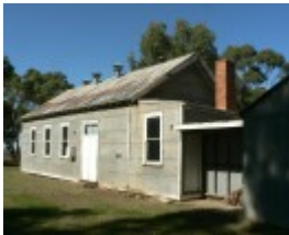
Gringegalgon Soldiers Memorial Hall - viewed from north-west
