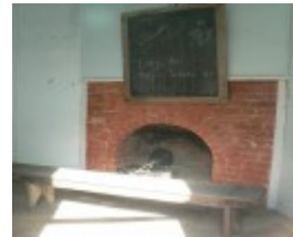
Gringegalgon Soldiers Memorial Hall - rear dressing room
