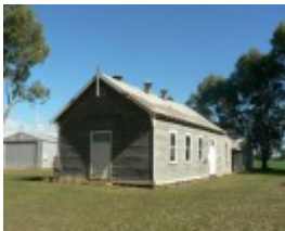
Gringegalgon Soldiers Memorial Hall - viewed from north-east
