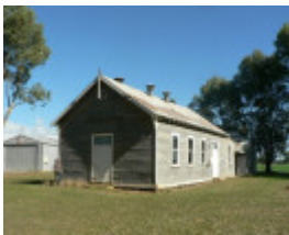
Gringegalgon Soldiers Memorial Hall - viewed from north-east
