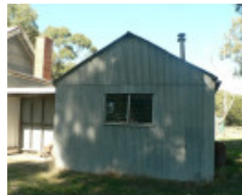
Gringegalgon Soldiers Memorial Hall - supper room/kitchen
