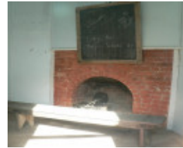
Gringegalgon Soldiers Memorial Hall - rear dressing room
