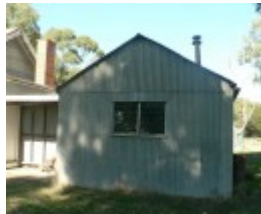
Gringegalgon Soldiers Memorial Hall - supper room/kitchen
