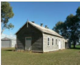
Gringegalgon Soldiers Memorial Hall - viewed from north-east
