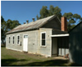
Gringegalgon Soldiers Memorial Hall - viewed from north-west
