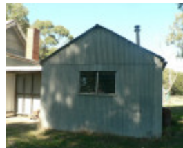
Gringegalgon Soldiers Memorial Hall - supper room/kitchen
