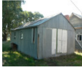
Gringegalgon Soldiers Memorial Hall - supper room/kitchen
