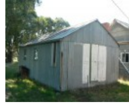
Gringegalgon Soldiers Memorial Hall - supper room/kitchen
