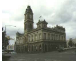
1 ballarat town hall exterior view 1993
