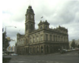
1 ballarat town hall exterior view 1993
