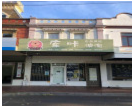
45-47 Waverley Road, Malvern East
