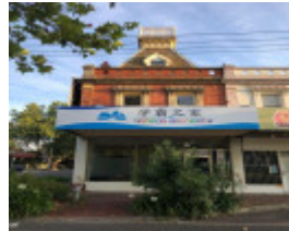
45-47 Waverley Road, Malvern East
