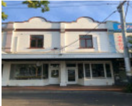
49-51 Waverley Road, Malvern East
