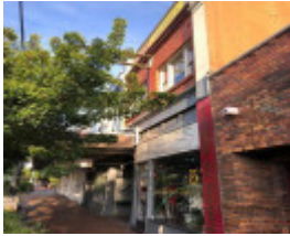
53-57 Waverley Road, Malvern East
