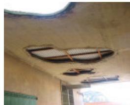
Maribyrnong substation cutouts in concrete roof
