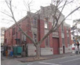
Carlton tram substation front and west side
