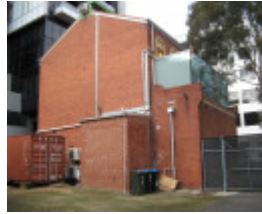
South Yarra tram substation rear view
