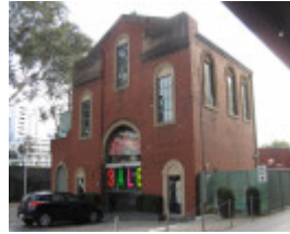
South Yarra tram substation
