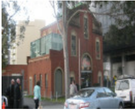
Tram substation Sth Yarra 5 Sep 2012 KJ (1).JPG
