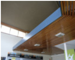
Interior of primary entrance building - timber panelling
