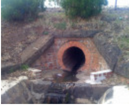
Railway culvert, Station Street
