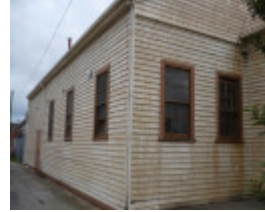
PROGRESS HALL SIDE ELEVATION
