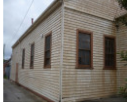
PROGRESS HALL SIDE ELEVATION
