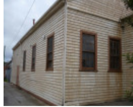
PROGRESS HALL SIDE ELEVATION
