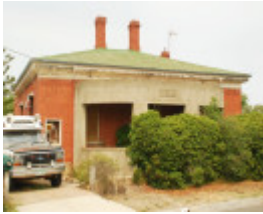
FORMER KAHLAND WINERY & CELLARS SOHE 2008
