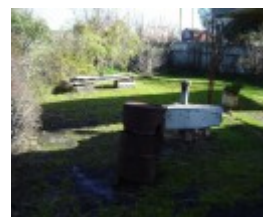
h02087 kahlands winery bendigo air vent 02 aug2005 mz
