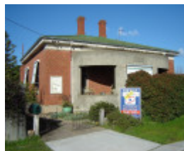
h02087 kahlands winery bendigo house exterior aug2005 mz
