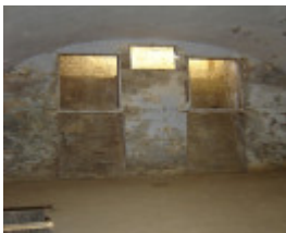
h02087 kahlands winery bendigo air vent 03 aug2005 mz
