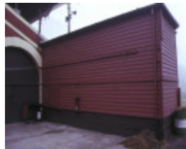
queen elizabeth oval grandstand bendigo entrance
