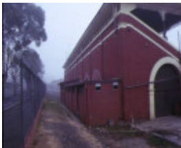
queen elizabeth oval grandstand bendigo rear view
