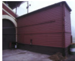
queen elizabeth oval grandstand bendigo entrance
