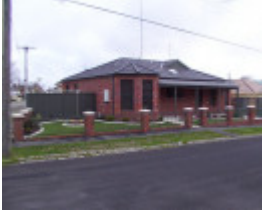
10 Steinfeld Street South
