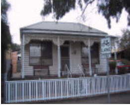
204 Peel Street North
