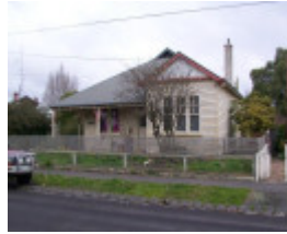
26 Steinfeld Street South
