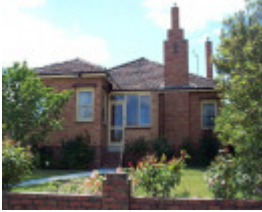
806 Lydiard Street North
