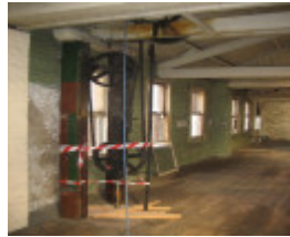
61-9 A'Beckett St lift first floor MZ 24 05 2007
