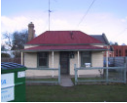
15 Otway Street North
