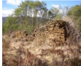
H0070 lyrebird gully hop kiln bagging room
