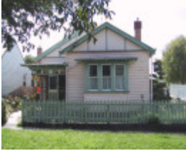
415 Talbot Street South
