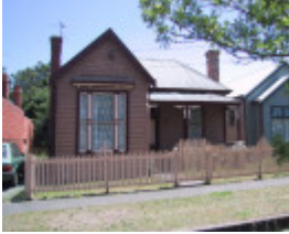
426 Raglan Street South
