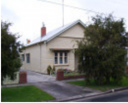
31- Anderson Street East
