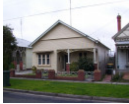
31- Anderson Street East
