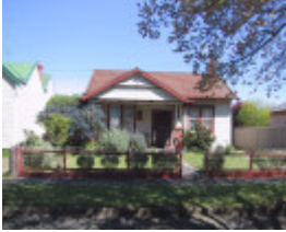
514 Talbot Street South
