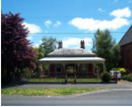
413 Lydiard Street North
