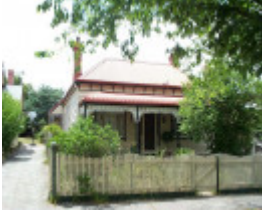
510 Lydiard Street North
