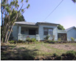
411 Peel Street North
