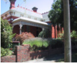
6 Raglan Street South
