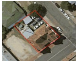
Donald Offices - Aerial 2023
