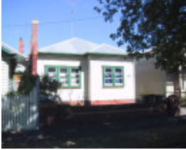
218 Raglan Street South
