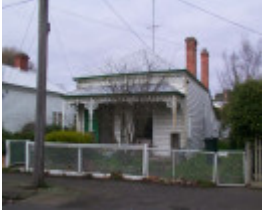
42 Steinfeld Street South
