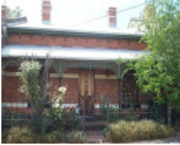
422 Lydiard Street North
