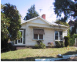
401 Peel Street North
