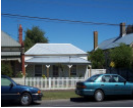
619 Lydiard Street North
