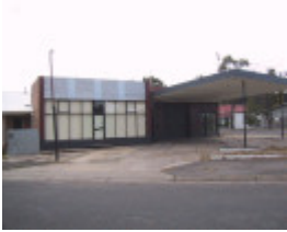
303 Peel Street North
