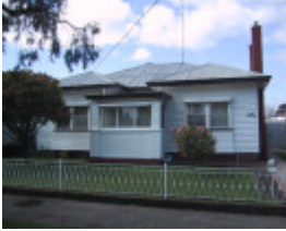
212 Peel Street North
