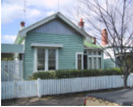
216 Peel Street North
