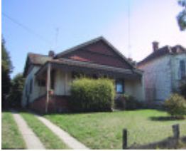
403 Peel Street North
