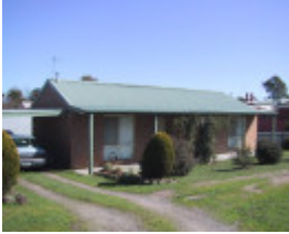
21 King Street North
