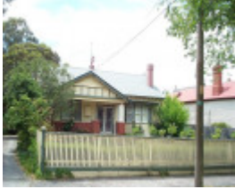
512 Lydiard Street North
