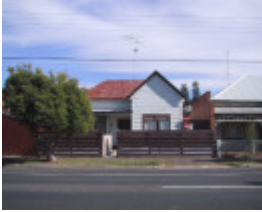
305 Peel Street North
