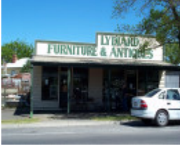
205-207photo01 Lydiard Street North
