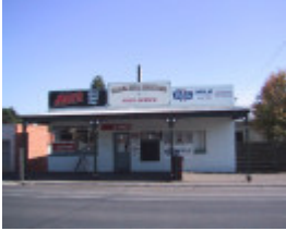
503 Peel Street North
