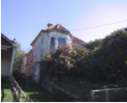
405 Peel Street North
