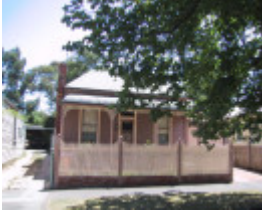
306 Raglan Street South
