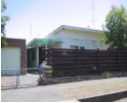
402 Raglan Street South
