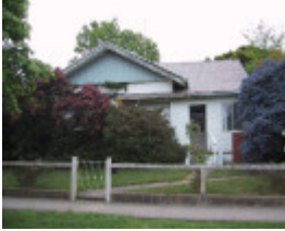
201 Ripon Street South
